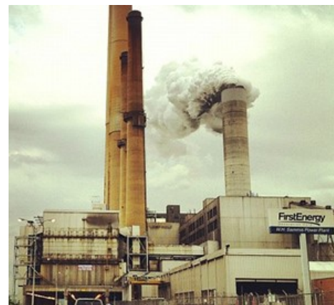
W.H. Sammis plant Source: FirstEnergy
